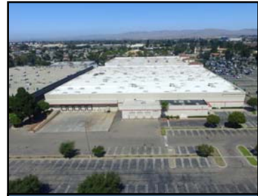
Former Costco Building Santa Maria, CA 1335 South Bradley Rd. Bldg Type: Commercial Bldg Size: 132,108 SF Lot Size: 8.48 AC Acquired: Aug 2021
