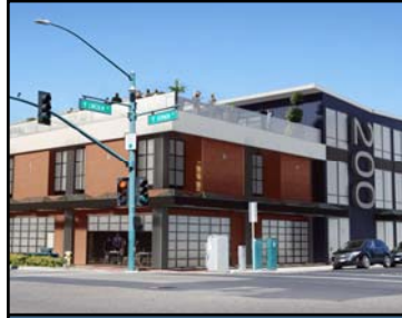
200 Vernon Building Sacramento, CA 200 Vernon St. Bldg Type: Redevelopment Bldg Size: 40,000 SF Lot Size: 0.696 AC Acquired: Nov 2021
