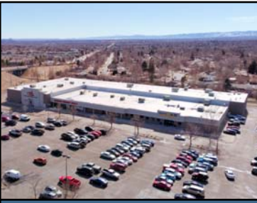
Neighborhood Shopping Cntr Westminster, CO 8601 Sheridan Blvd. Bldg Type: Commercial Bldg Size: 71,367 SF Lot Size: 6.295 AC Acquired: Jul 2021
